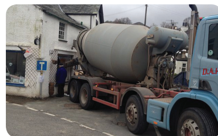
Cement being poured into the shop.
